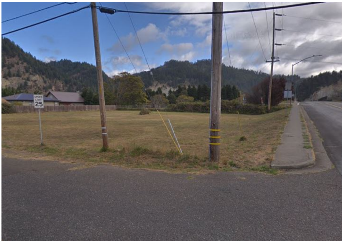
Figure 6: Sidewalk Terminates at the intersection of Davis St. and Ireland St. (No crosswalk or ADA ramps)
