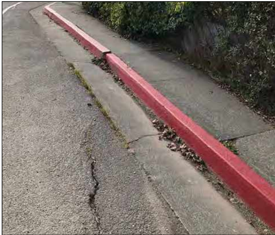
Photo 2. Surface Failure Along Alignment (Storm Drain Improvement #1)
