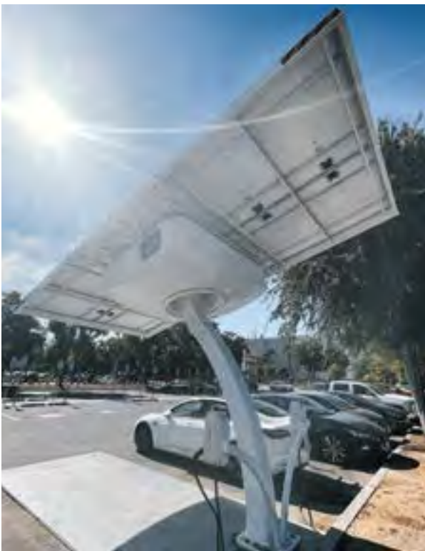
Figure 9: Solar Charging Station
