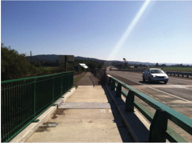
Photo 7 Bridge railing on Highway 101 over the Mad River, Humboldt County
