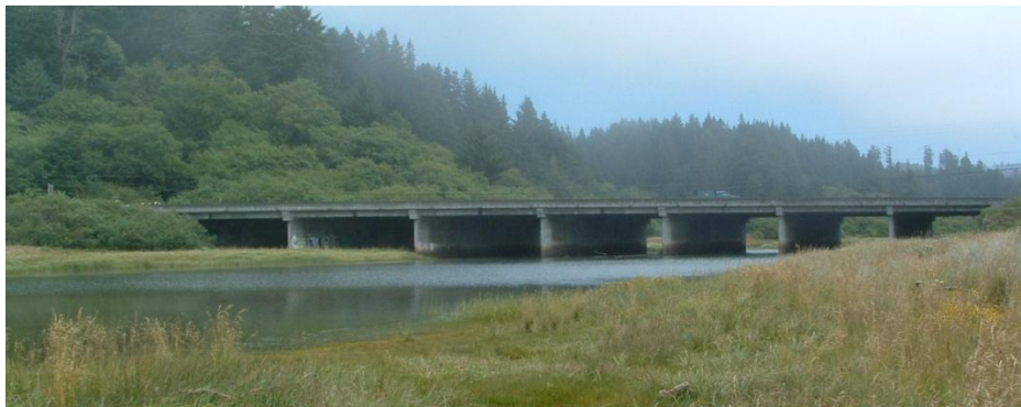
Highway 101 Bridge Over the Little River - Overall View
