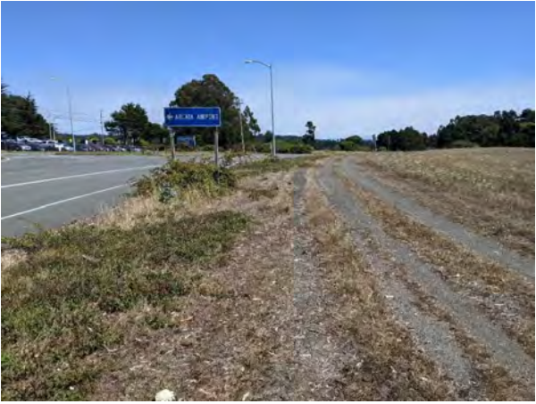
Photo 6. Abandoned Road Grade along Airport Road. Could this be a trail?
