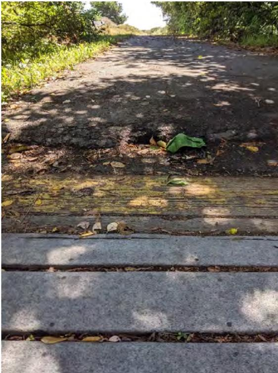
**Photo 2. Strawberry Creek Bridge South Footing. Wood or rubber ramp needed.**
