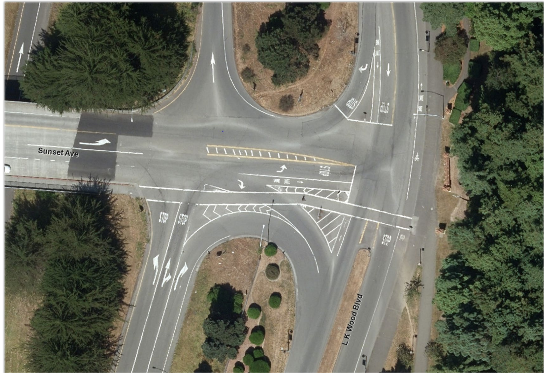
Figure 2.1 The current configuration of the two intersections located within the project area. The Sunset Avenue/US 101 northbound ramp intersection is a four-legged intersection with the north and south leg acting as US 101 Northbound on- and off- ramps. The Sunset Avenue/LK Wood Boulevard is an all-way stop located 150 feet east of the Sunset Ave/US 101 northbound ramps intersection.
