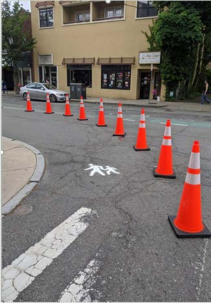
Above: Cones and a simple stencil were used to extend sidewalks in Somerville, MA
