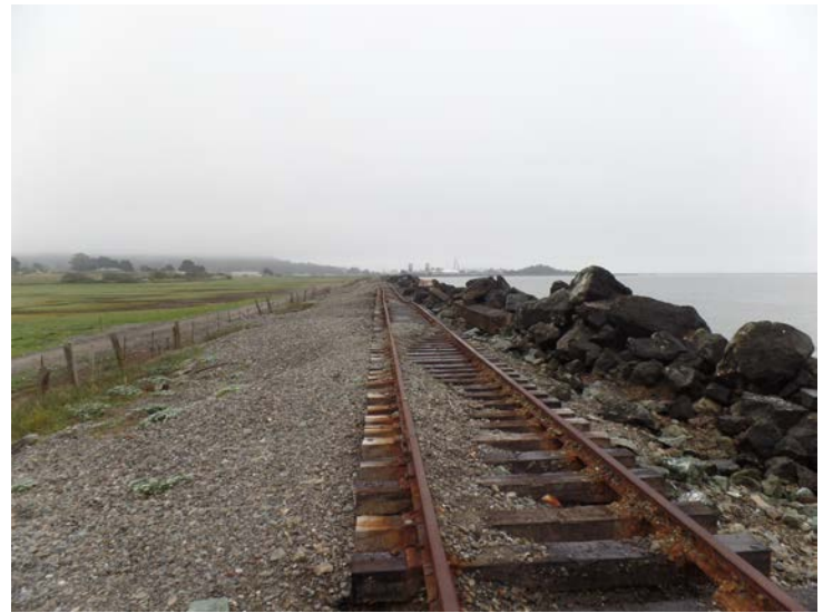
Existing NCRA right-of-way along Humboldt Bay
