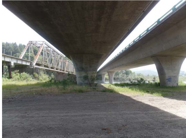
Highway 101 and NCRA bridges over Van Duzen River
