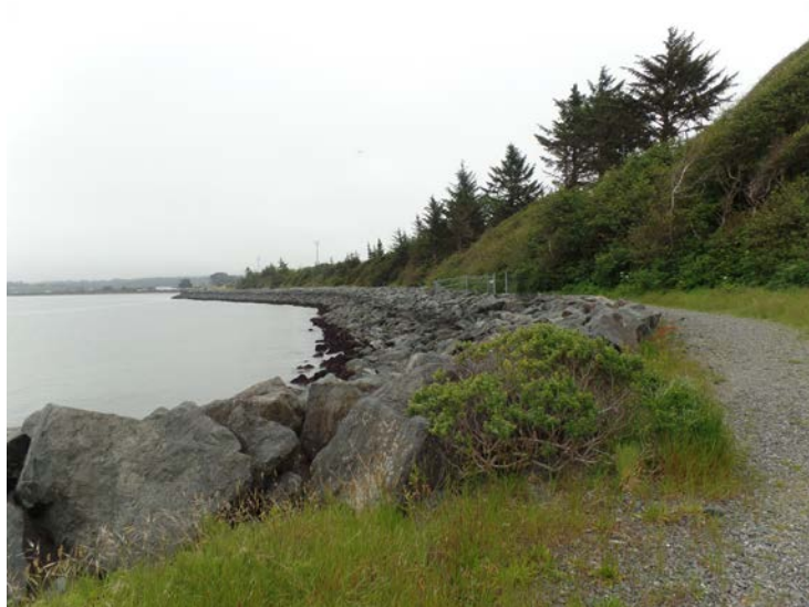
Existing public access path around PG&E property
