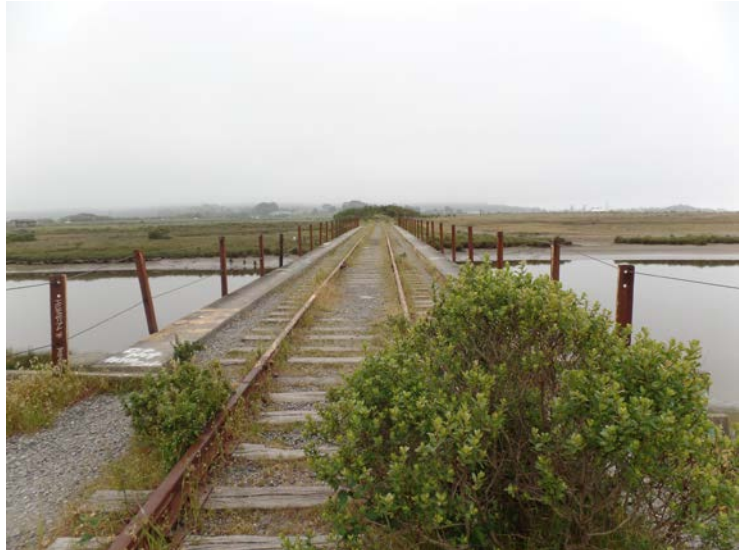
Existing NCRA Elk River crossing
