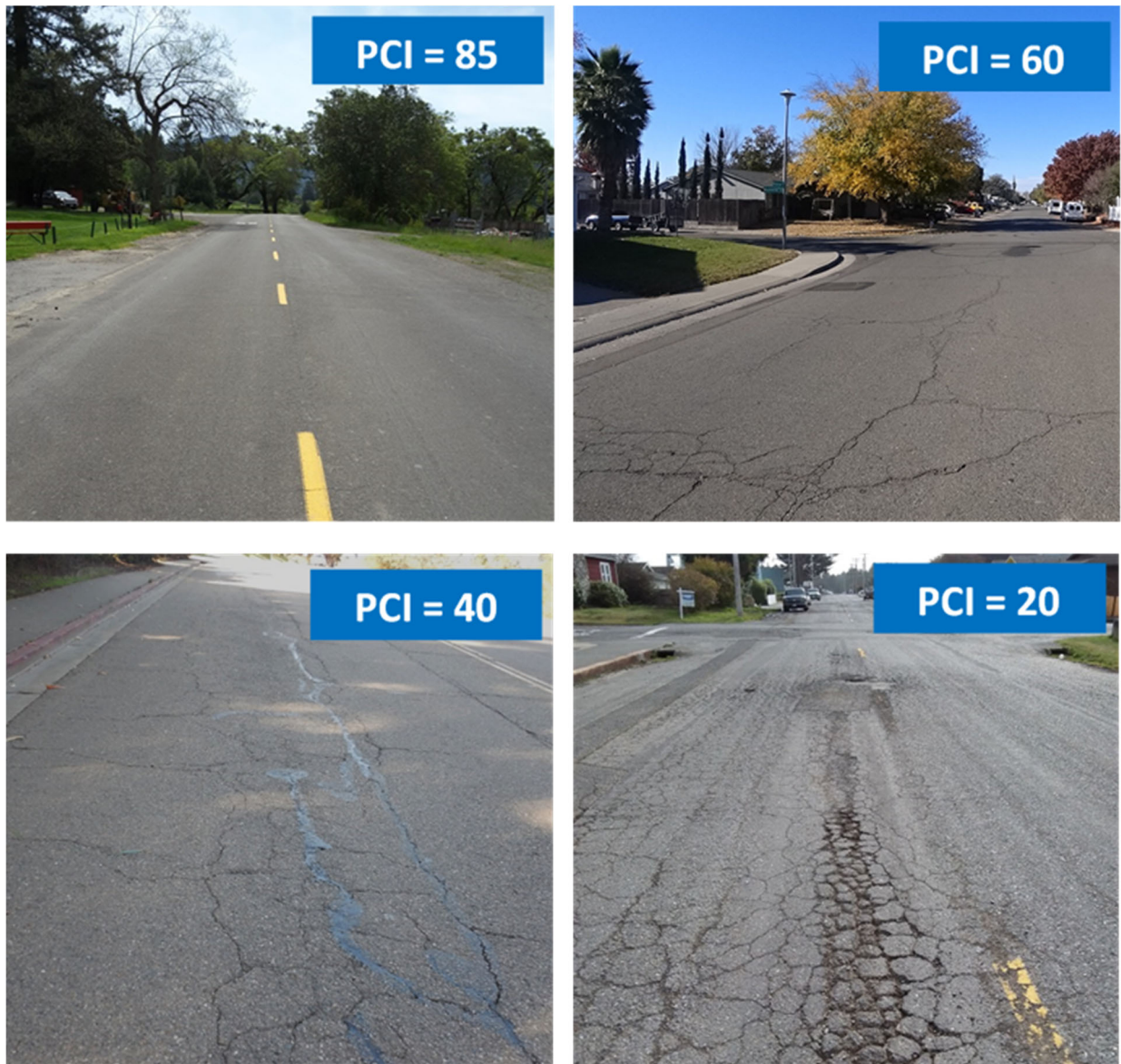
Figure 1. Examples of Streets with Different PCIs
