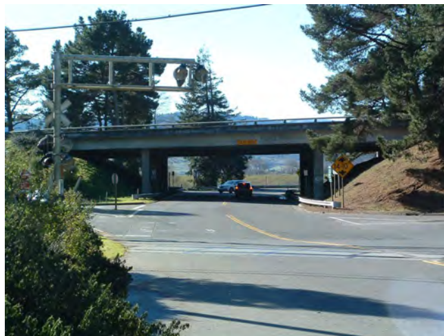
Kenmar Road Undercrossing Looking West
