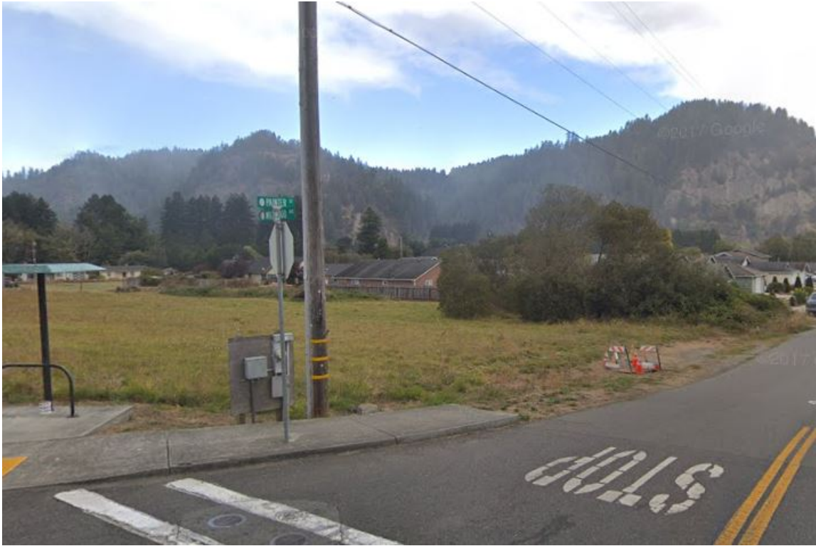
Figure 10: Sidewalk terminates at the intersection of Painter St. and Wildwood Ave.
