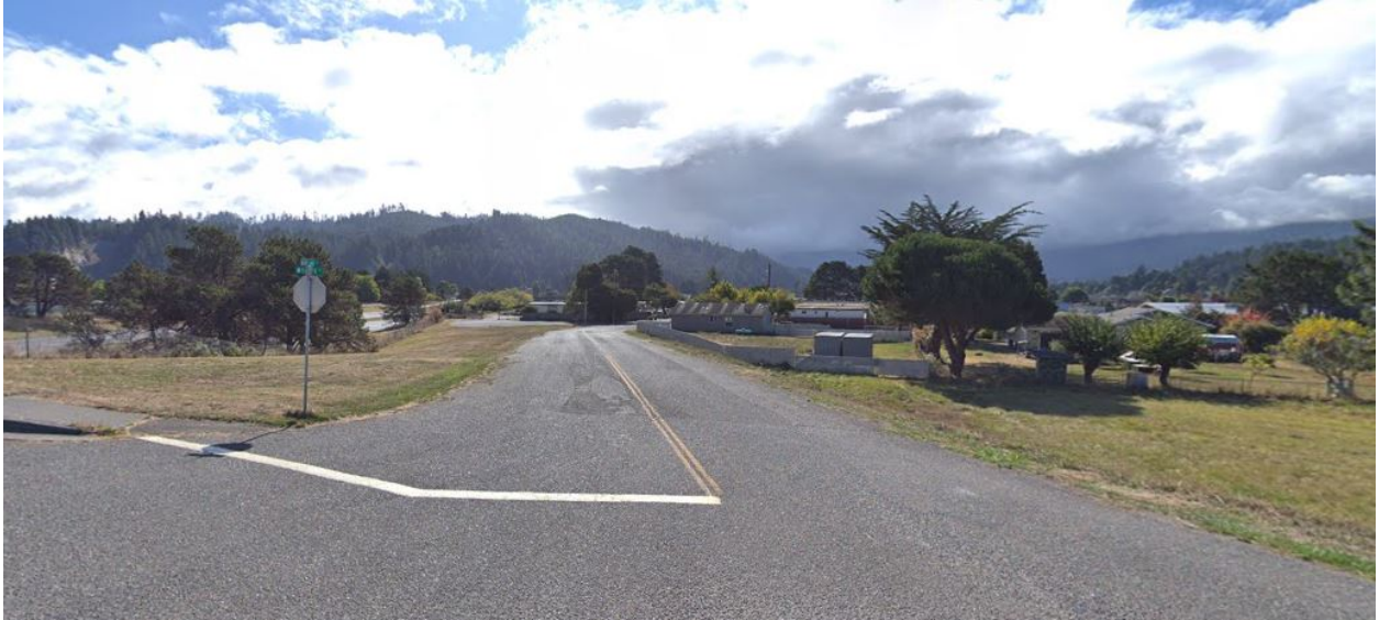
Figure 7: Missing sidewalk, ADA ramps and crosswalks at the southern intersection of Painter and Ireland
