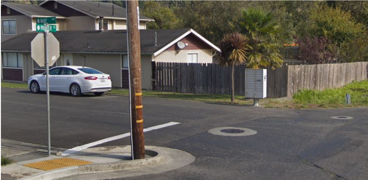
Figure 9: Missing sidewalk and ADA ramps at the intersection of Painter St. and May Ave.
