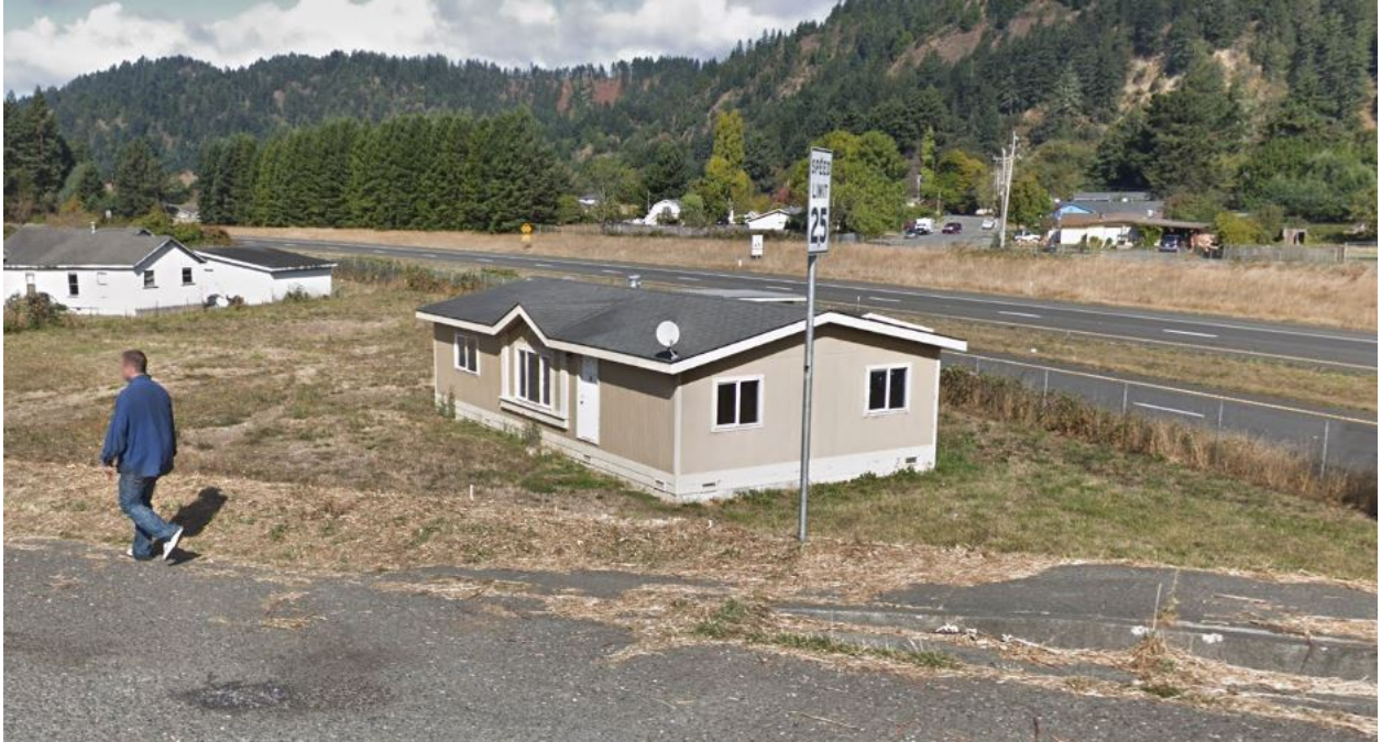
Figure 8: Existing sidewalk terminates and no cross walk or ADA ramp at the northern intersection of Painter St. and Ireland St.
