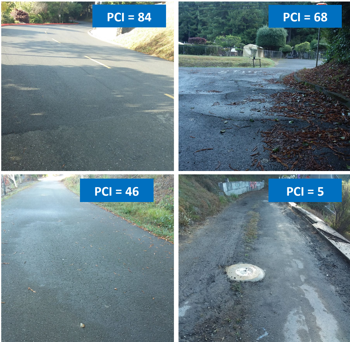
Figure 1. Examples of Roads with Different PCIs
