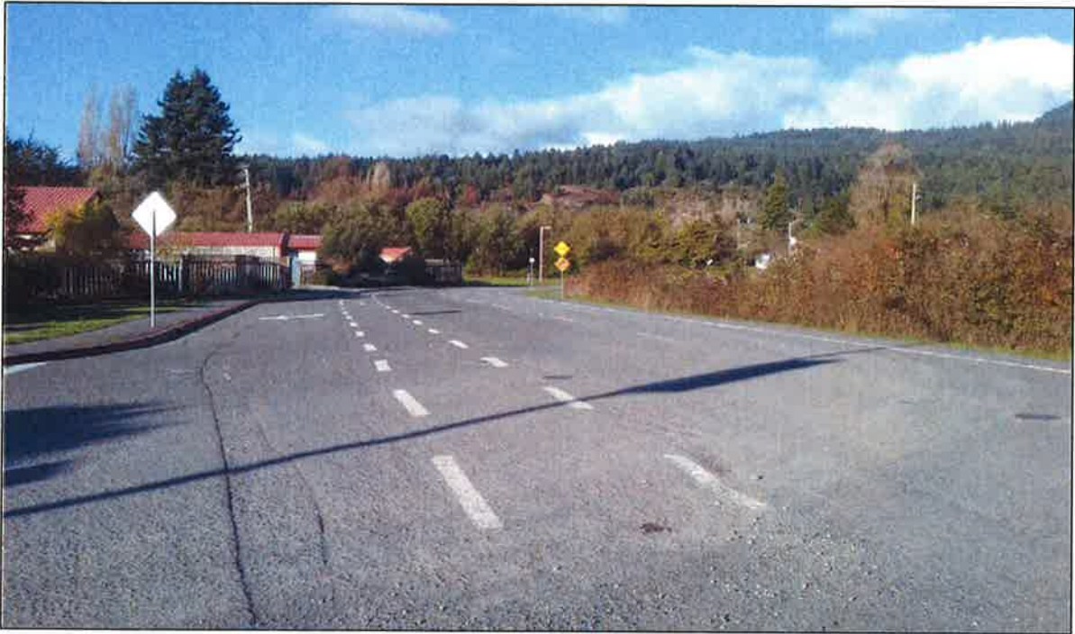
Hatchery Road and Taylor Way, looking north.
